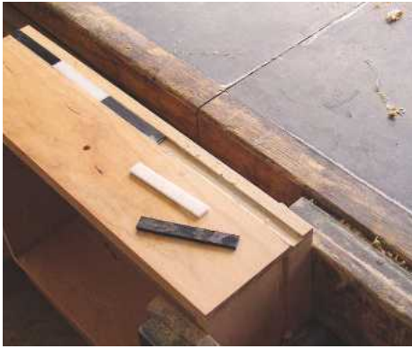
▲ Pic.19 The glass sections were glued into the routed grooves with builder's epoxy
